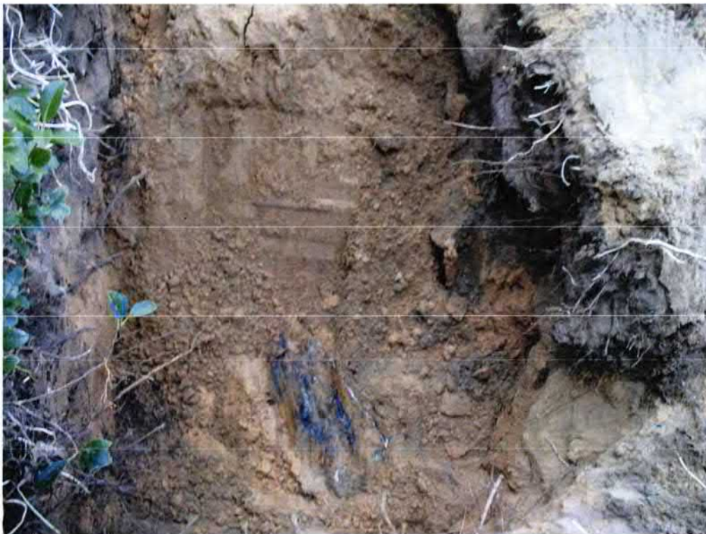
Picture 2: UST 885Cobia excavation in progress.
